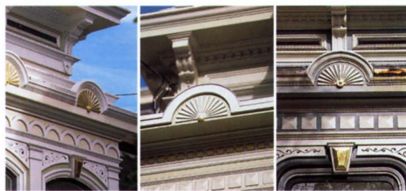
LEFT AND ABOVE: No architectural detailing on the Mevi home survived, so inspiration for replacement trim was borrowed from neighboring homes that line the shady block.
